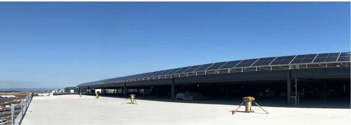
**The PDX Airport** solar awning extends 600ft along the parking structure and has a rated capacity of 75.2kW DC. Tigo dedicated rapid shutdown devices are installed on each of the 177x 400W Trina modules.
