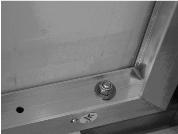
Figure 3 – Washer and Nut Placement Inside Module Frame
