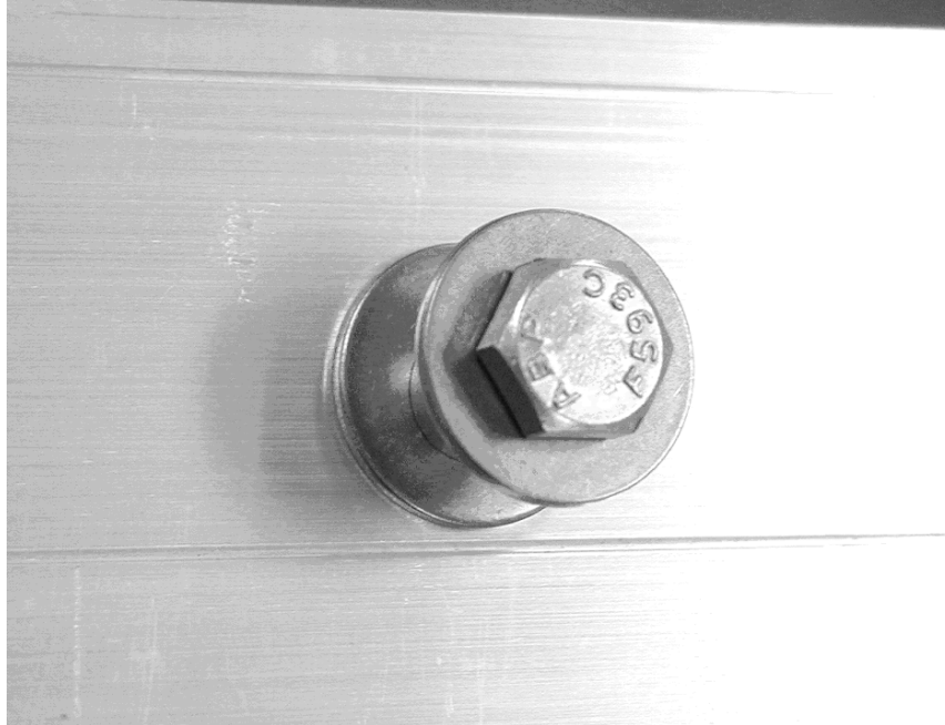
Figure 2 – Head of Mounting Pin Outside of Frame
