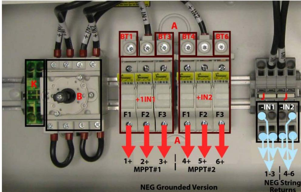
**Figure 2.06b- DC Array Connection**
