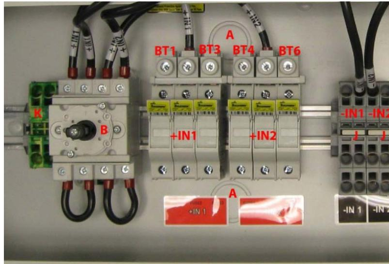
Figure 2.06a – DC Array Connection PVI-10.0-I-OUTD-S1-US/CAN-XXX-YY
