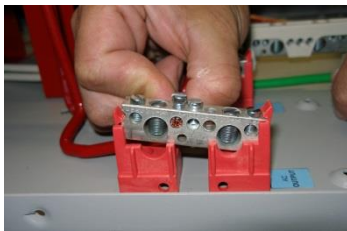
Finish removing the terminal block
