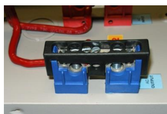
Replace wiring cover. Black cover shown here
