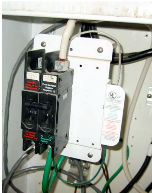
Figure 12. External Ground-Fault Protection Device
